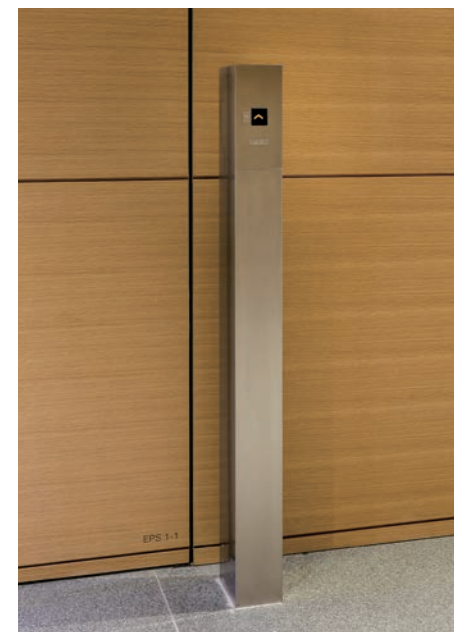
Hall button, 1st floor (the pole for hall button is installed by construction work)
