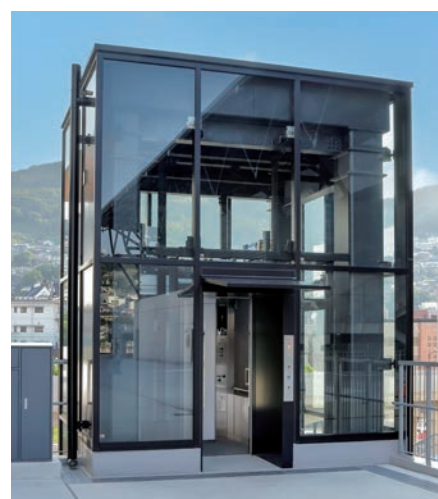
15-person passenger elevator, 3rd floor (concourse)
