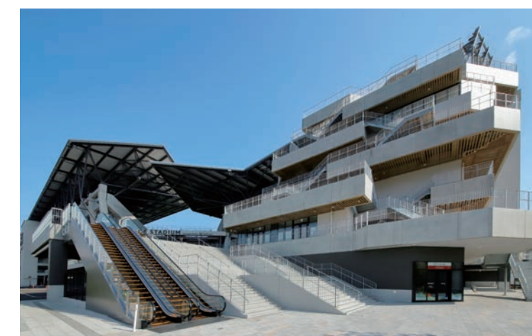
Escalator, 1th floor (Nagasaki Stadium City South)
