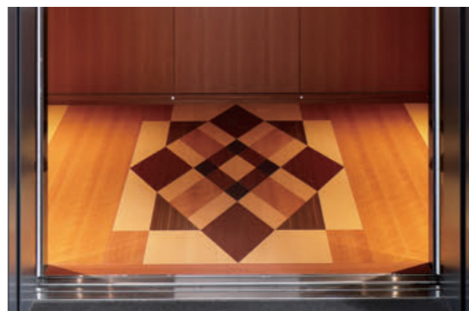
26-person passenger and freight (and emergency) elevator, elevator car floor (NOVARE Archives)
