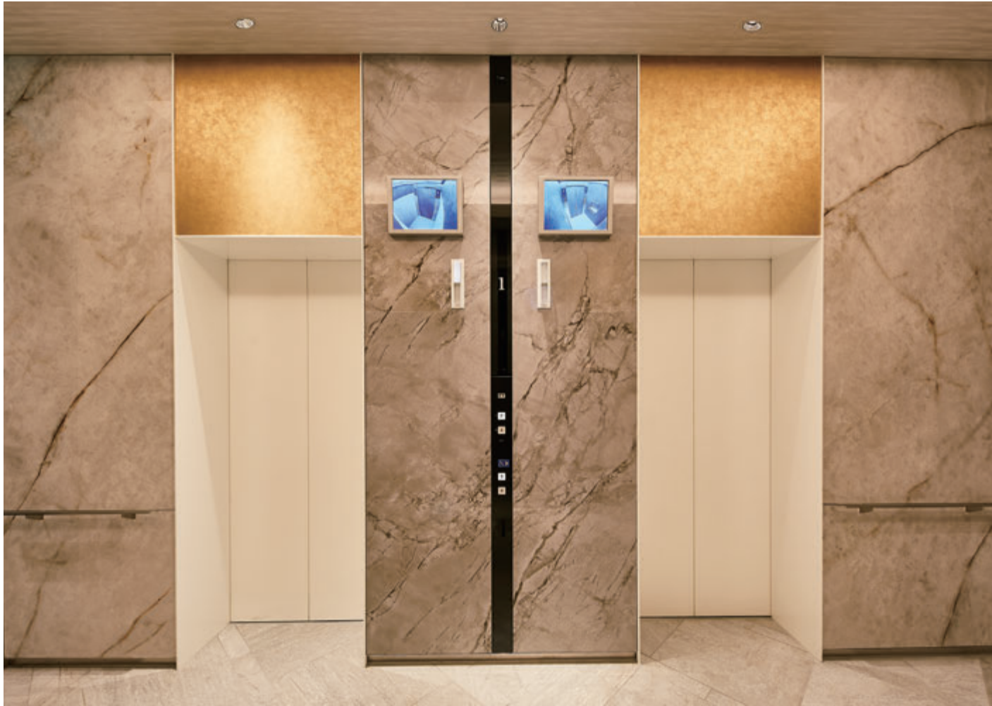
11-person passenger elevator, 1st floor (ONE Sapporo STATION Tower)
