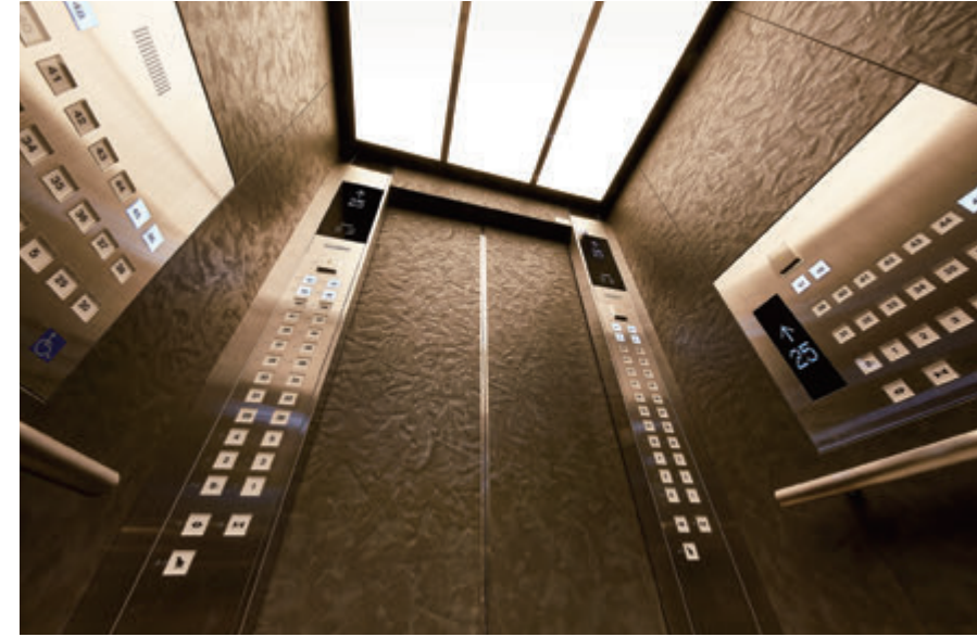
11-person passenger elevator, elevator car ceiling (ONE Sapporo STATION Tower)
