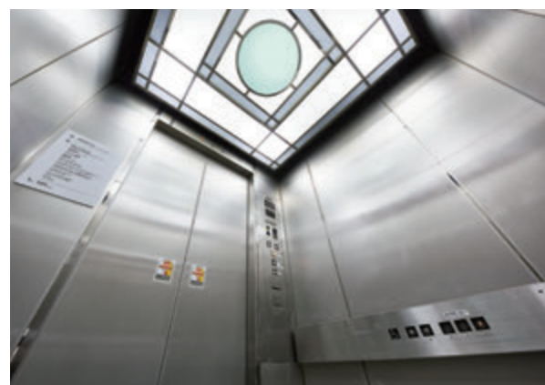
15-person passenger elevator, elevator car ceiling (before renovation)
