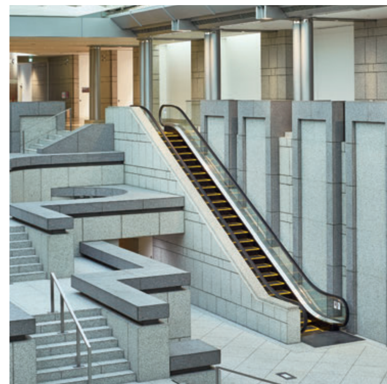
Escalator (after renovation)
