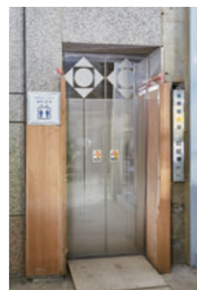
15-person passenger elevator, 2nd floor (before renovation)
