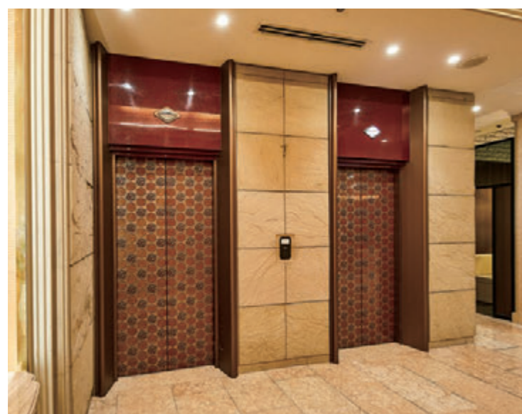
15-person passenger elevator, 1st floor hall (hall buttons, after renovation)
