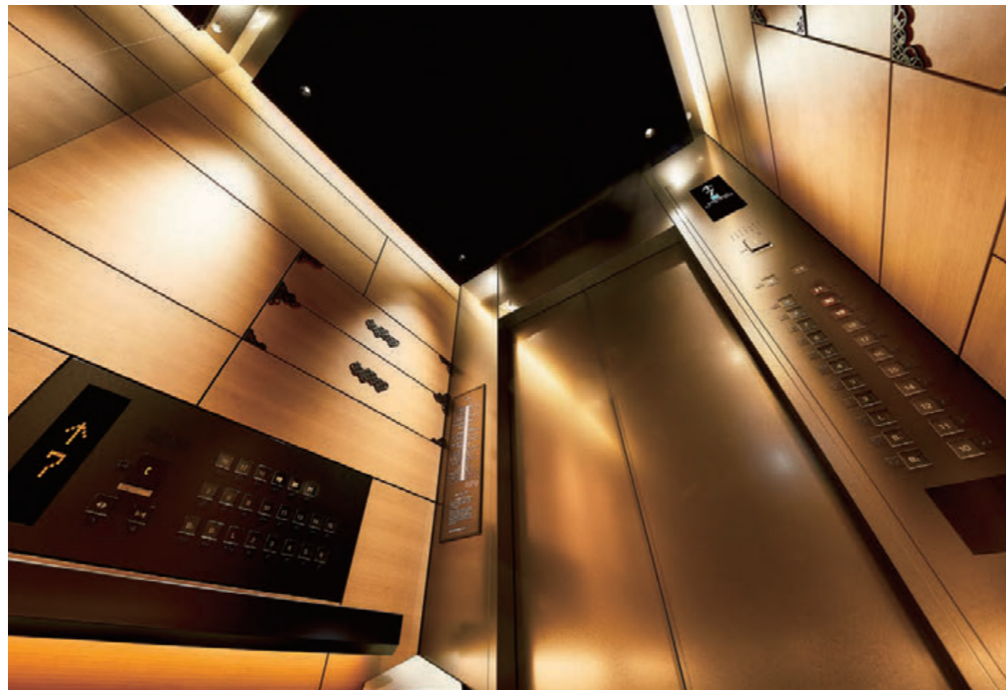
15-person passenger elevator, elevator car ceiling (after renovation)
