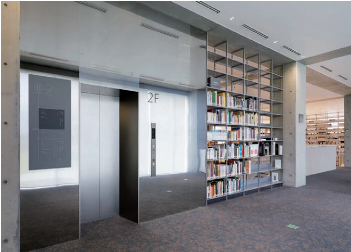
11-person passenger elevator, 2nd floor
