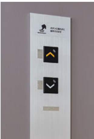
Elevator hall buttons (contact-free buttons)
