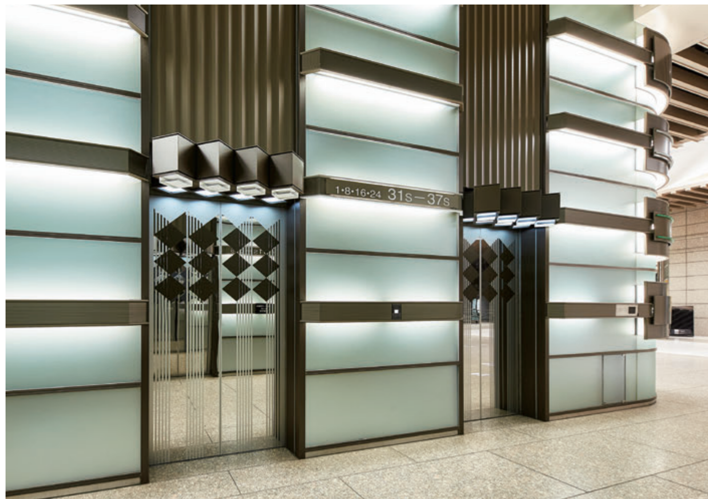
24-person passenger elevator, 1st floor (S Wing upper floor elevator bank, after renovation) The hall doors were also renovated based on the original design when the building was first completed.
