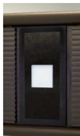
24-person passenger elevator, hall button (after renovation)
