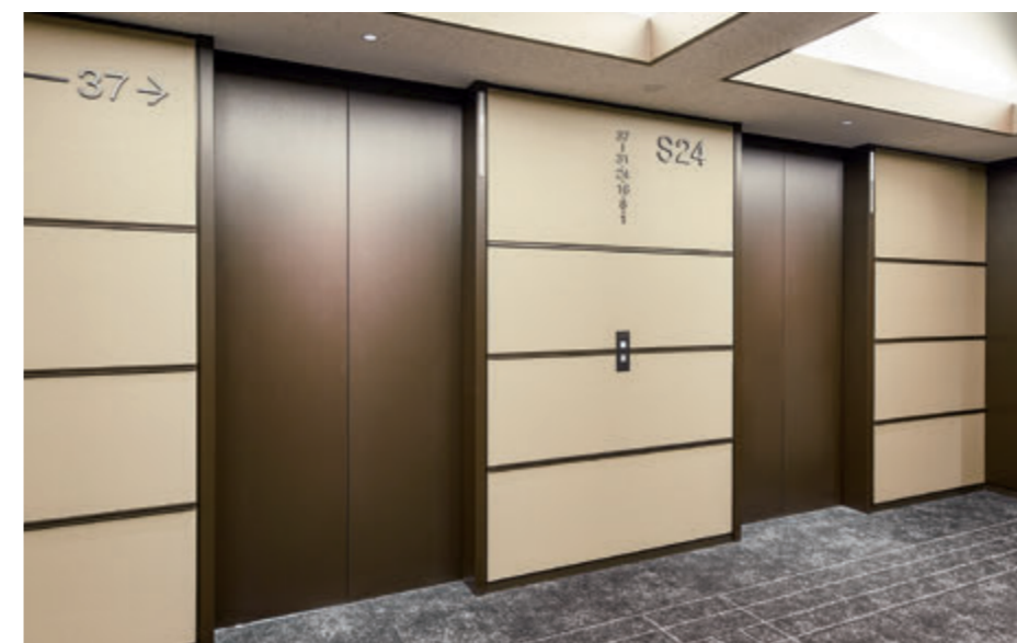
24-person passenger elevator, 24th floor hall (S Wing upper floor elevator bank, after renovation)
