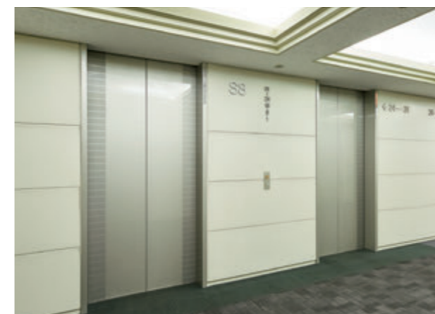
24-person passenger elevator, 8th floor hall (S Wing mid-floor elevator bank, before renovation)
