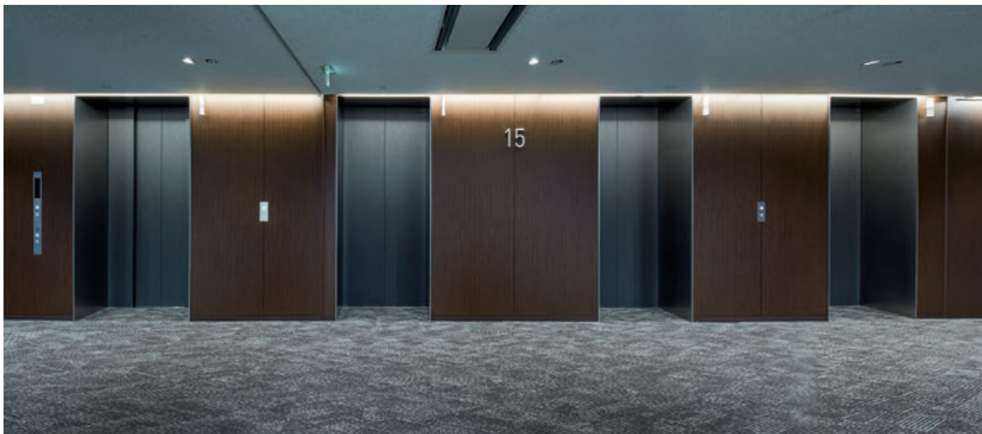
30-person passenger elevator, 15th floor
