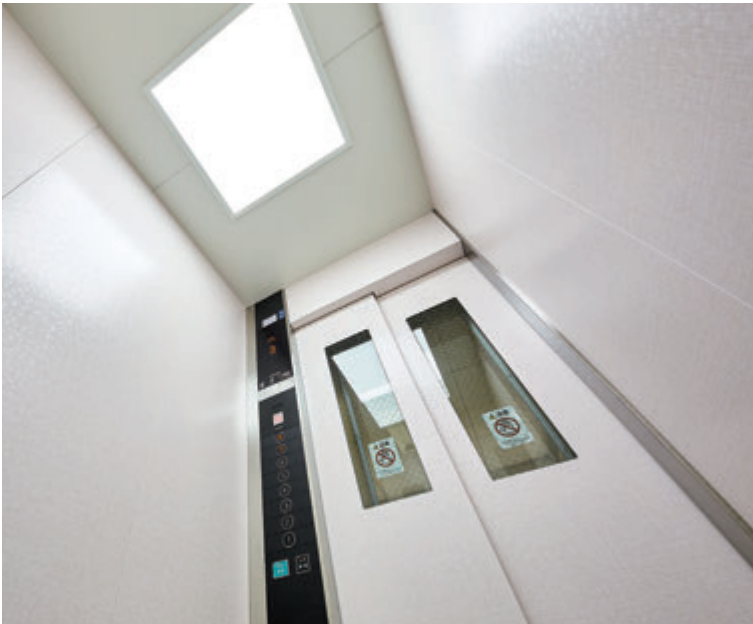
9-person (and trunk) residential elevator, elevator car ceiling (after renovation)
