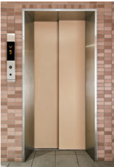
9-person (and trunk) residential elevator, 1st floor hall (after renovation)
