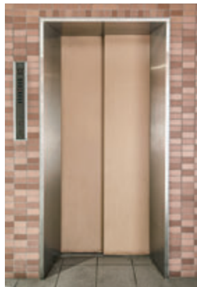
9-person (and trunk) residential elevator, 1st floor hall (before renovation)
