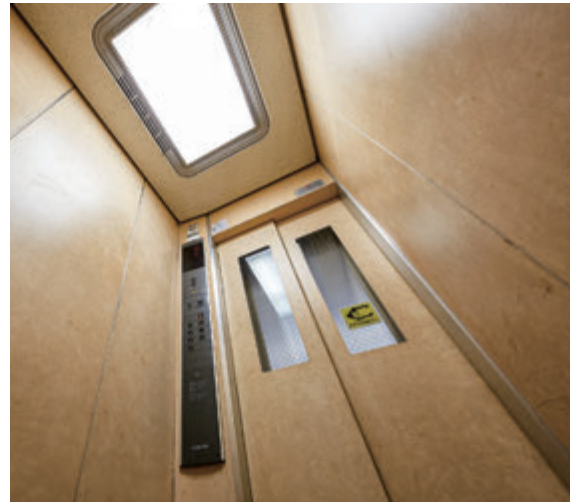
9-person (and trunk) residential elevator, elevator car ceiling (before renovation)
