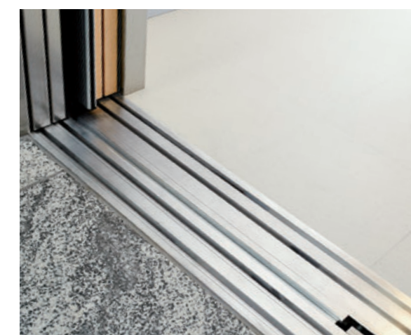
"Gap-free elevator design" fills gap between building and elevator
