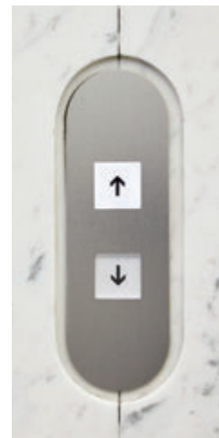
Elevator hall buttons (after renovation)
