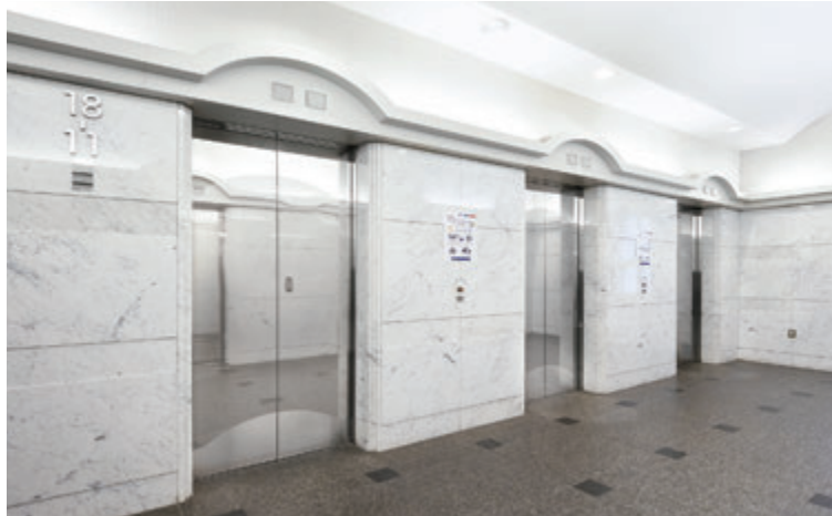
20-person passenger elevator, 1st floor hall (before renovation)
