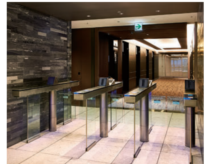
Destination floor selection system integrated with security gate, 25th floor office entrance
