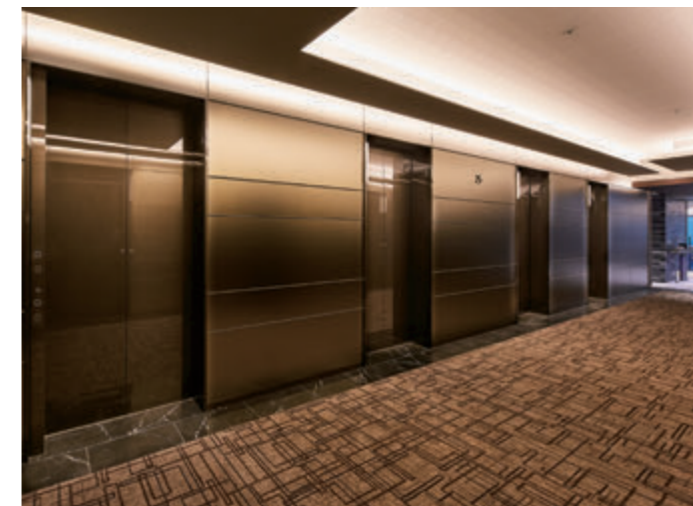
27-person and 24-person passenger elevators, 25th floor hall
