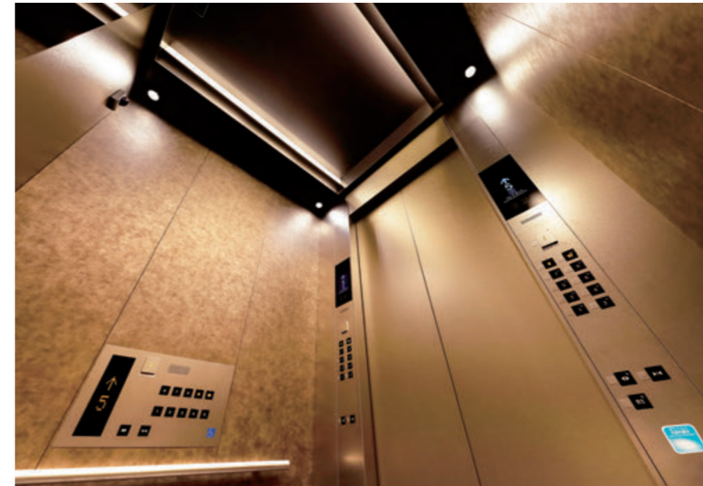
20-person passenger elevator, elevator car ceiling
