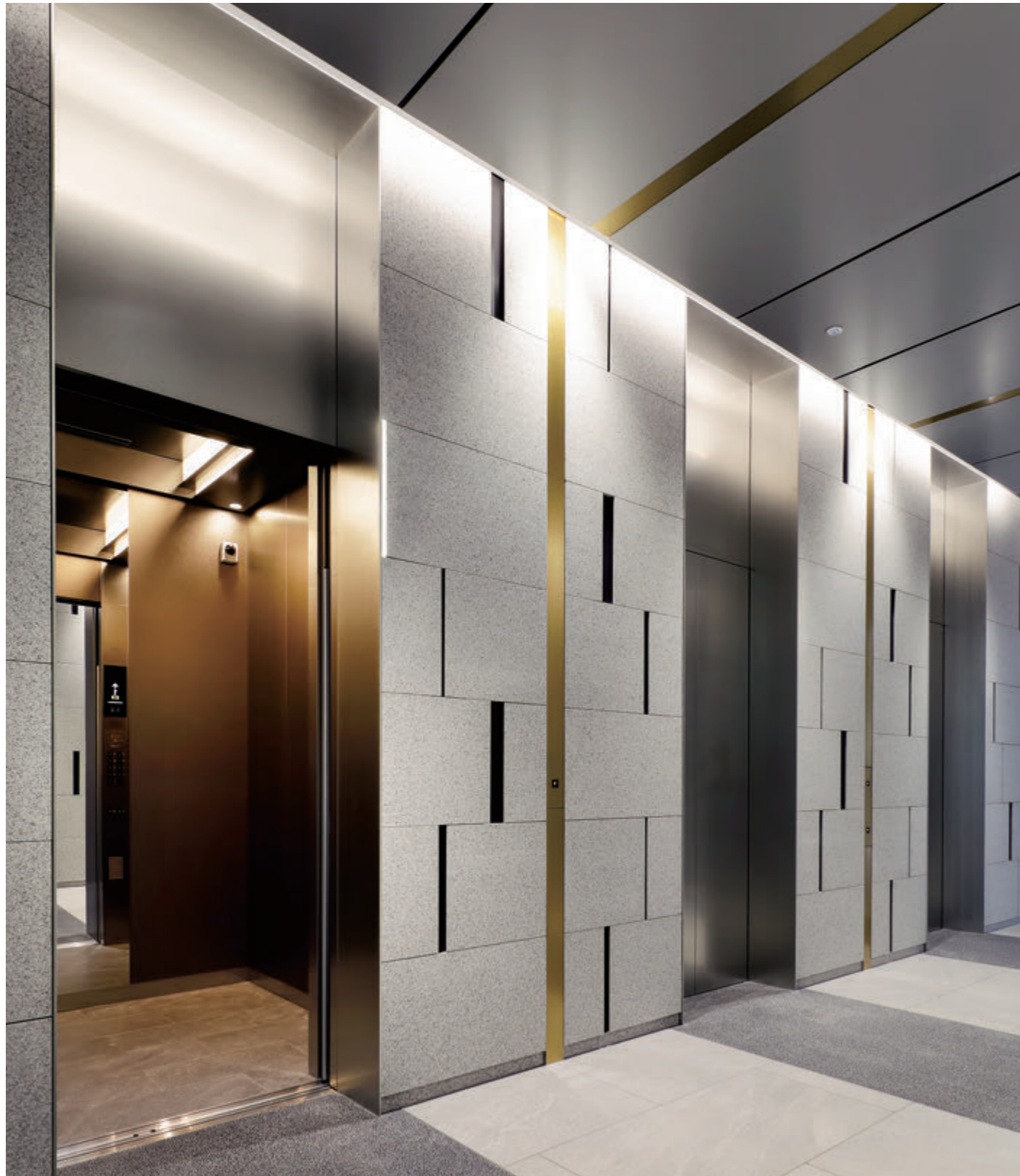
20-person passenger elevator, 1st floor hall
