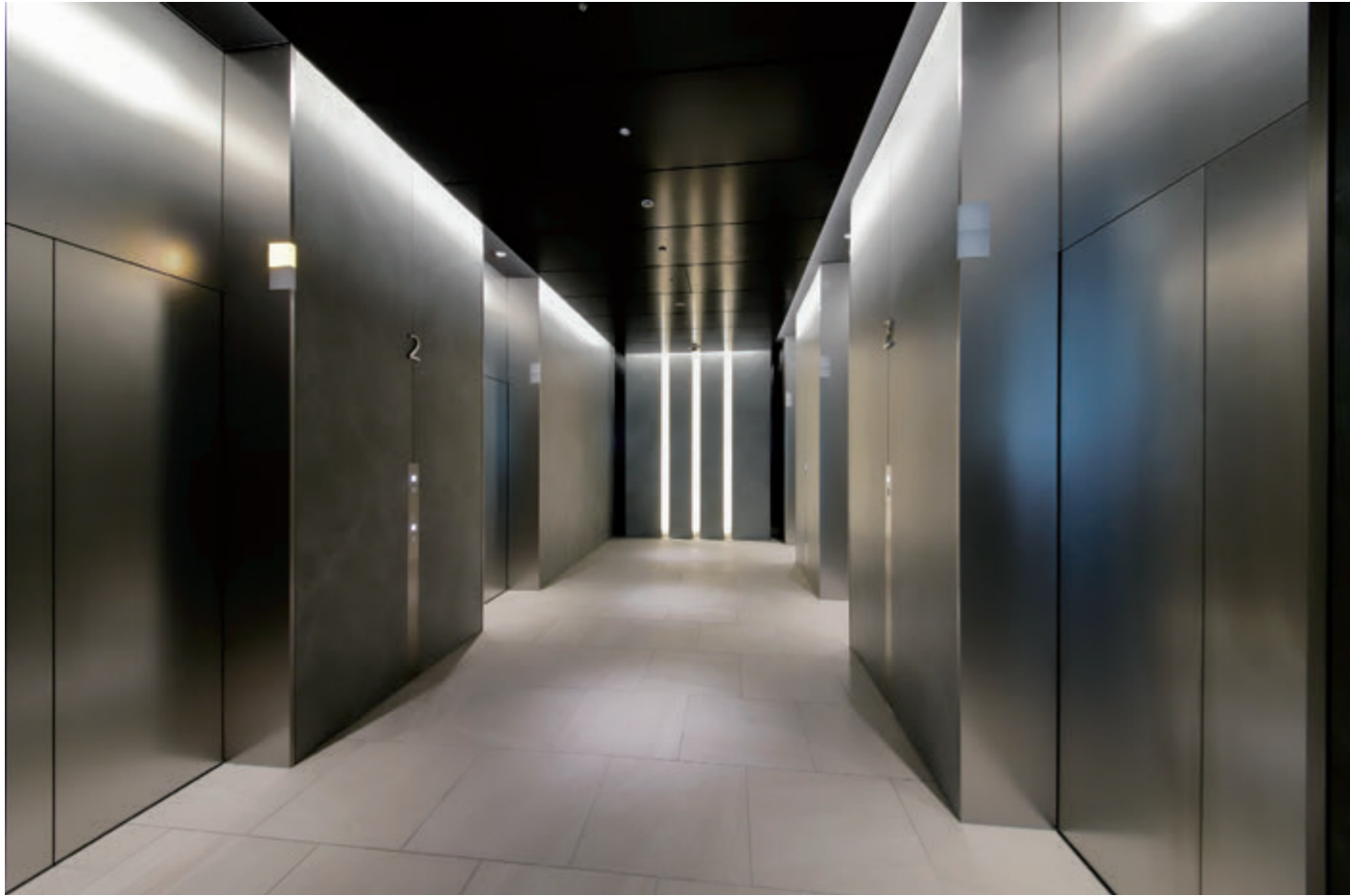
20-person passenger elevator, 1st floor hall
