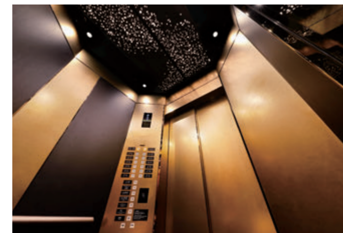
15-person passenger (observation) elevator, elevator car ceiling (after renovation)
