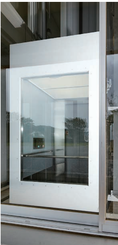
15-person passenger (observation) elevator, elevator car exterior
