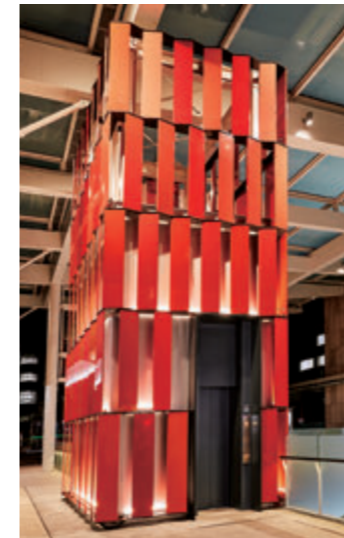
13-person passenger elevator, elevator shaft (Furumachi Rufuru Plaza)
