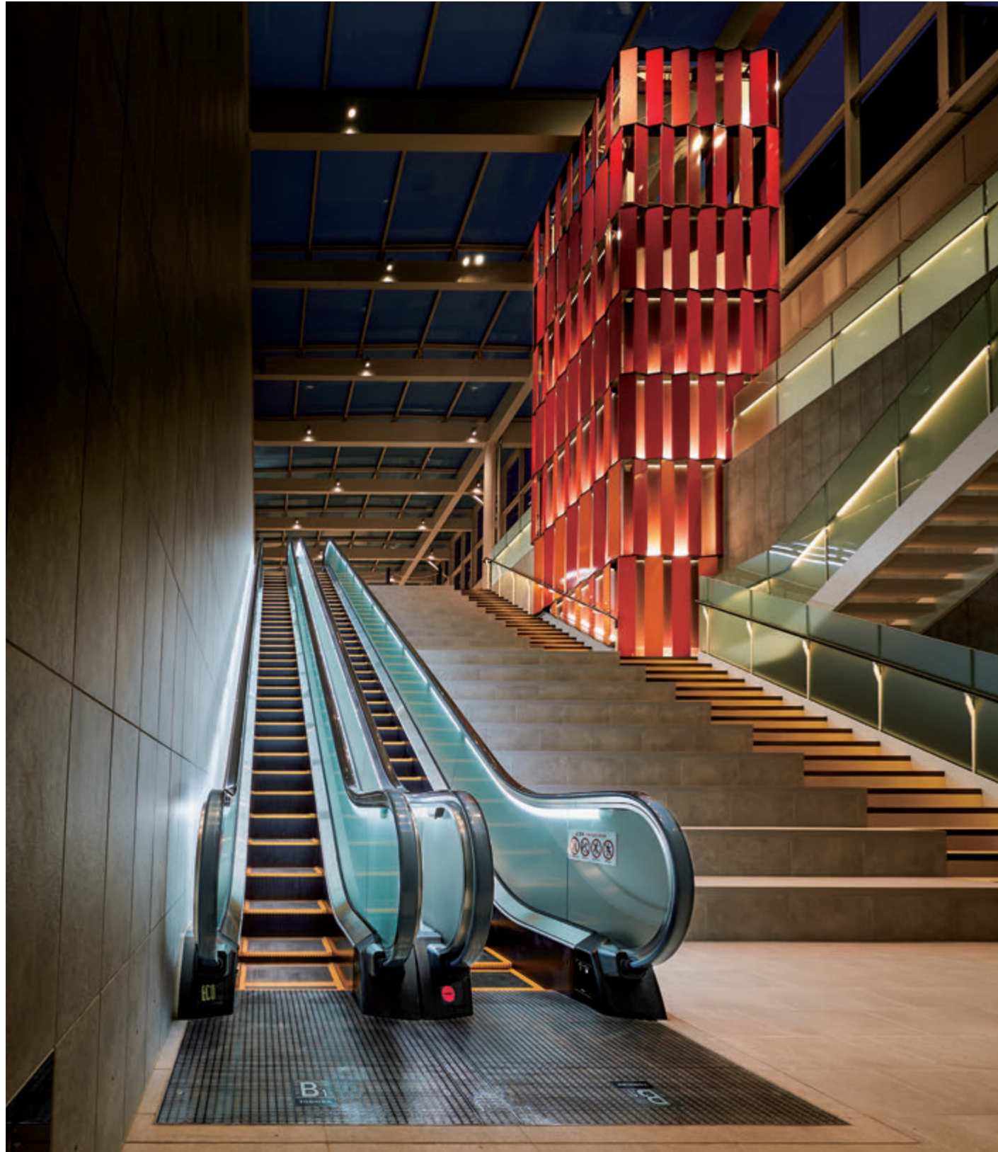
13-person passenger elevator, elevator shaft and escalator (Furumachi Rufuru Plaza)
