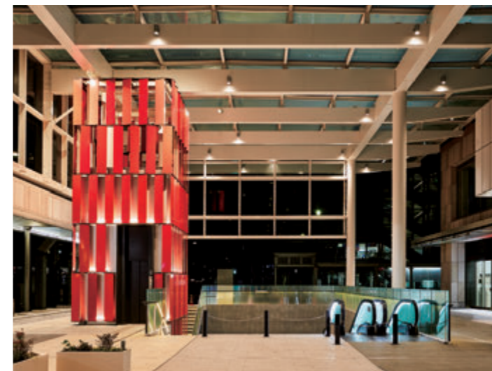
13-person passenger elevator, elevator shaft and escalator (Furumachi Rufuru Plaza)
