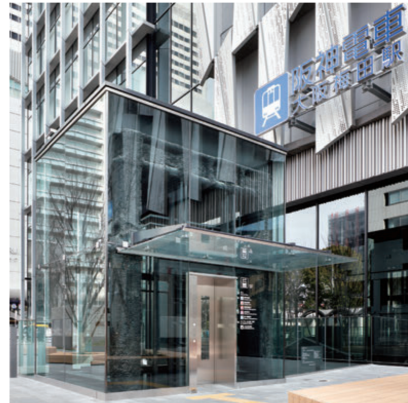
20-person passenger elevator, 1st floor
