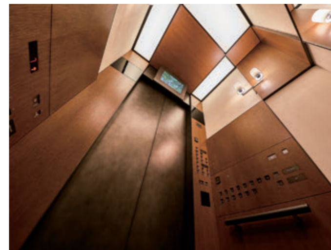
13-person passenger elevator, elevator car ceiling
