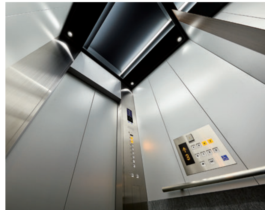
13-person passenger elevator, elevator car ceiling (after renovation to accommodate passengers in wheelchairs)
