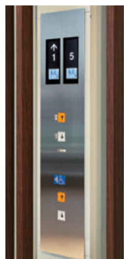
Elevator hall LCD indicator buttons, 1st floor (after renovation)
