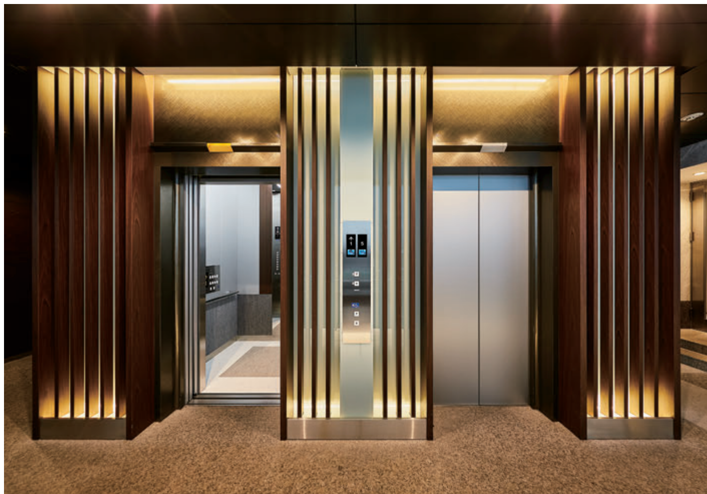
13-person passenger elevator, 1st floor hall (after renovation)
