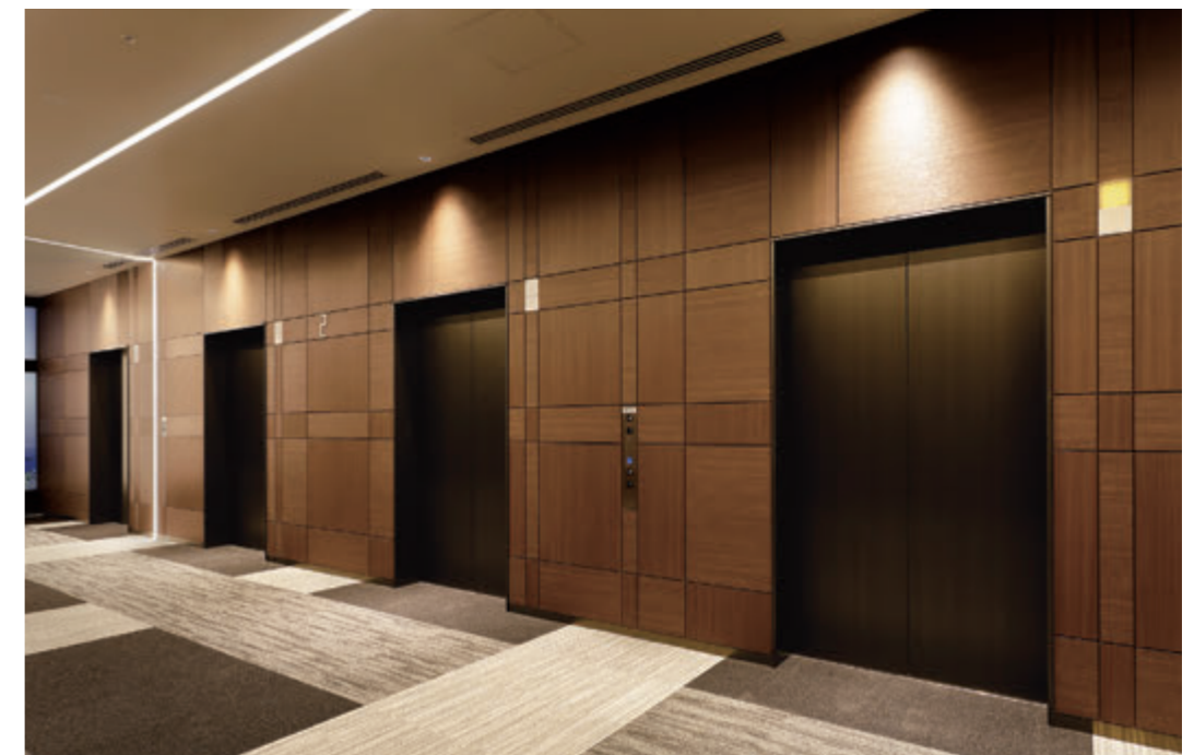
24-person passenger elevator, 2nd floor hall
