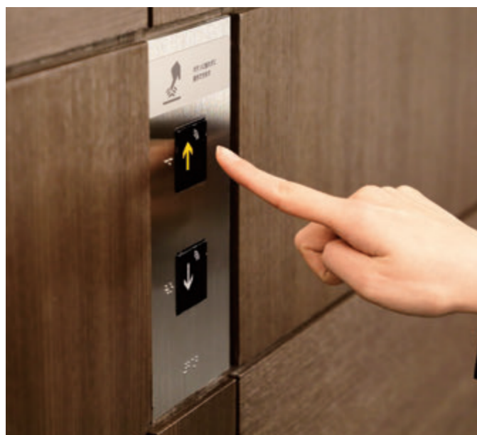
24-person passenger elevator, elevator hall control panel (contact-free buttons)
