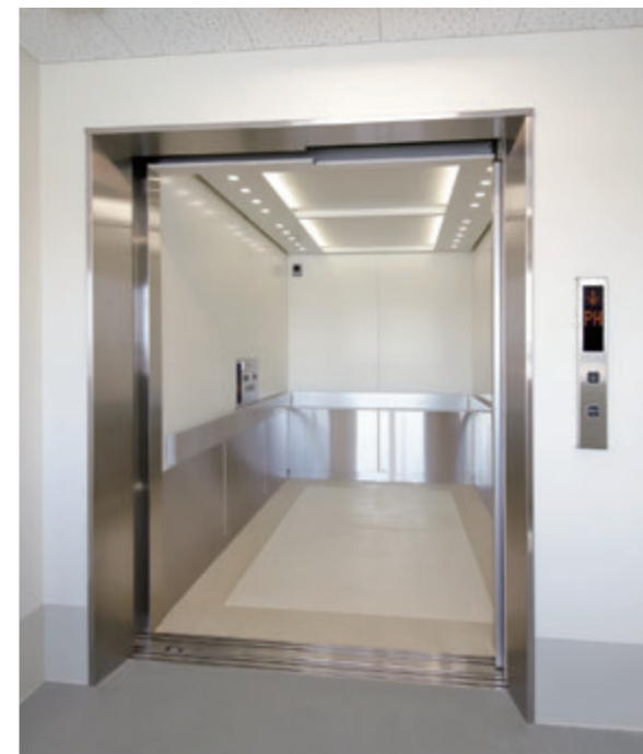
20-person hospital bed elevator, elevator car (heliport floor)
