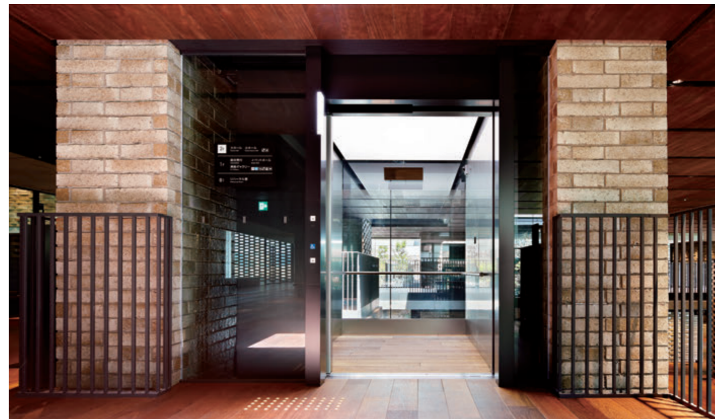
26-person passenger (observation) elevator, 2nd floor lobby
