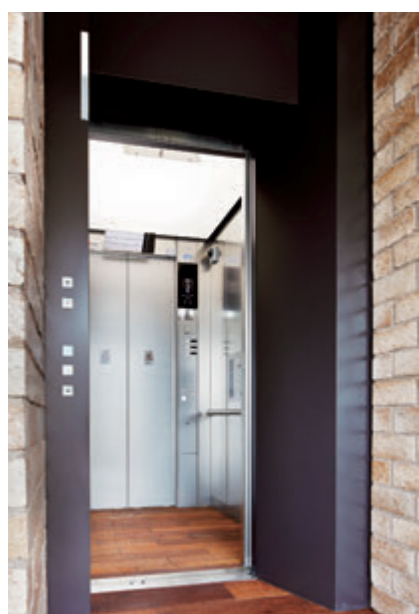
11-person passenger elevator, 3rd floor landing
