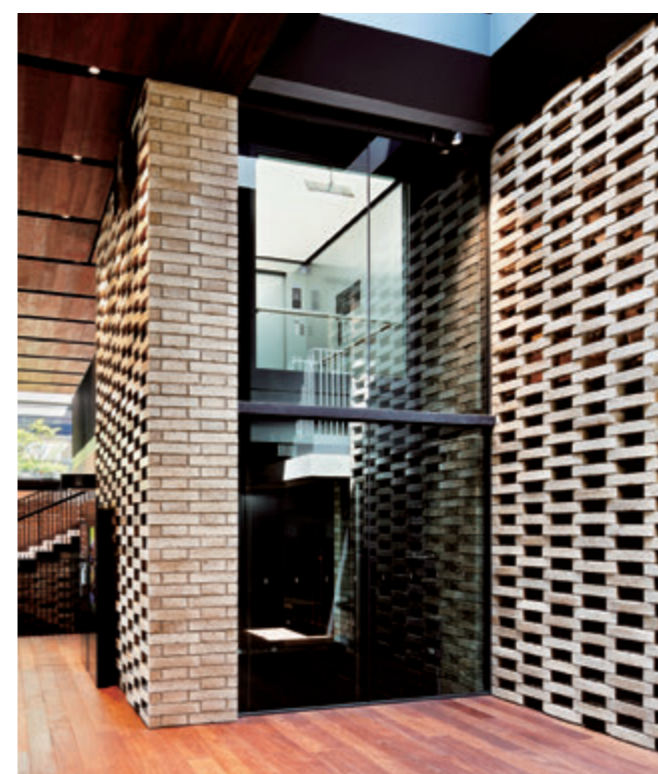
26-person passenger (observation) elevator, elevator shaft
