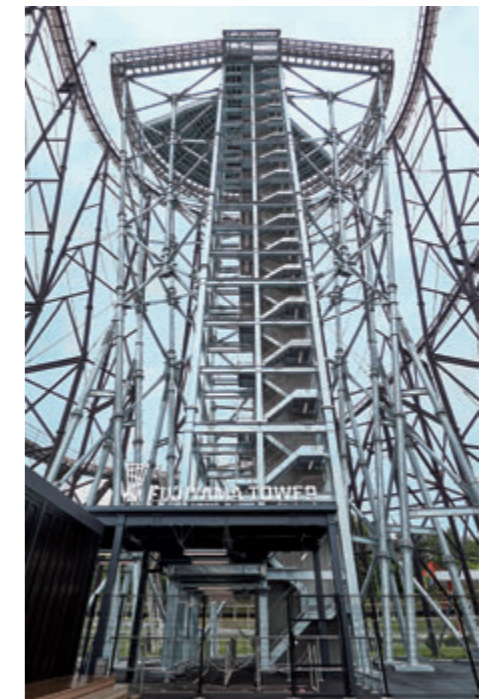
FUJIYAMA Tower (elevator shaft)
