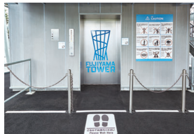
24-person passenger elevator, 1st floor landing
