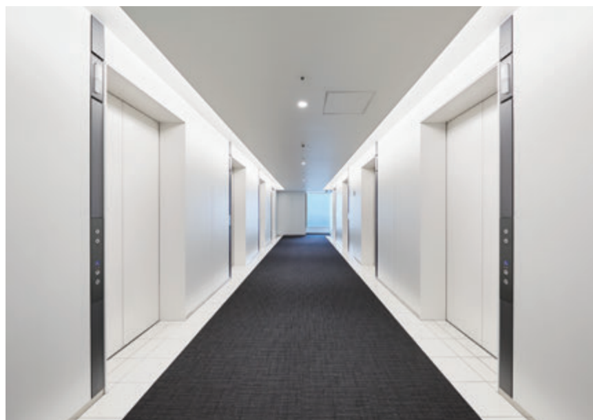
27-person passenger elevator, 28th floor hall
