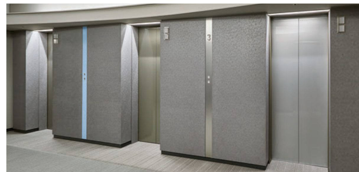
24-person passenger elevator, 3rd floor landing (right: after renewal, middle and left: before renewal)
