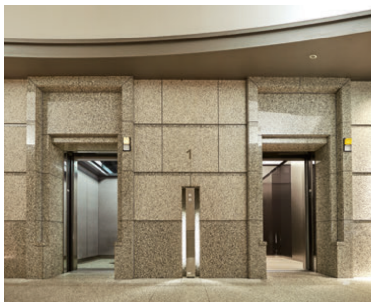
24-person passenger elevator, 1st floor hall (left: (before renewal, right: after renewal)
