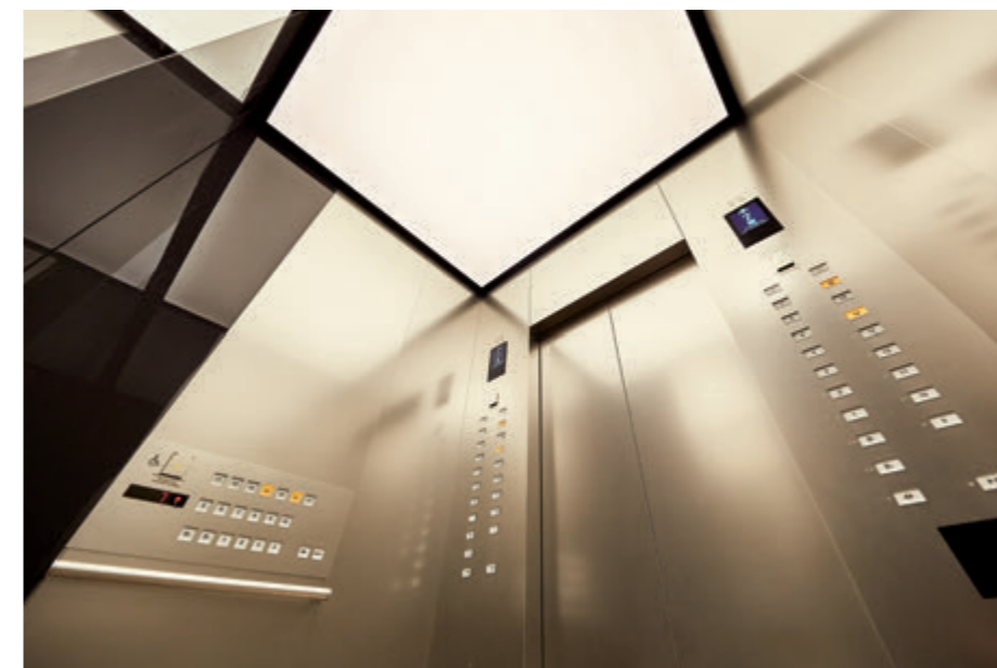
24-person passenger elevator car ceiling (after renewal)
