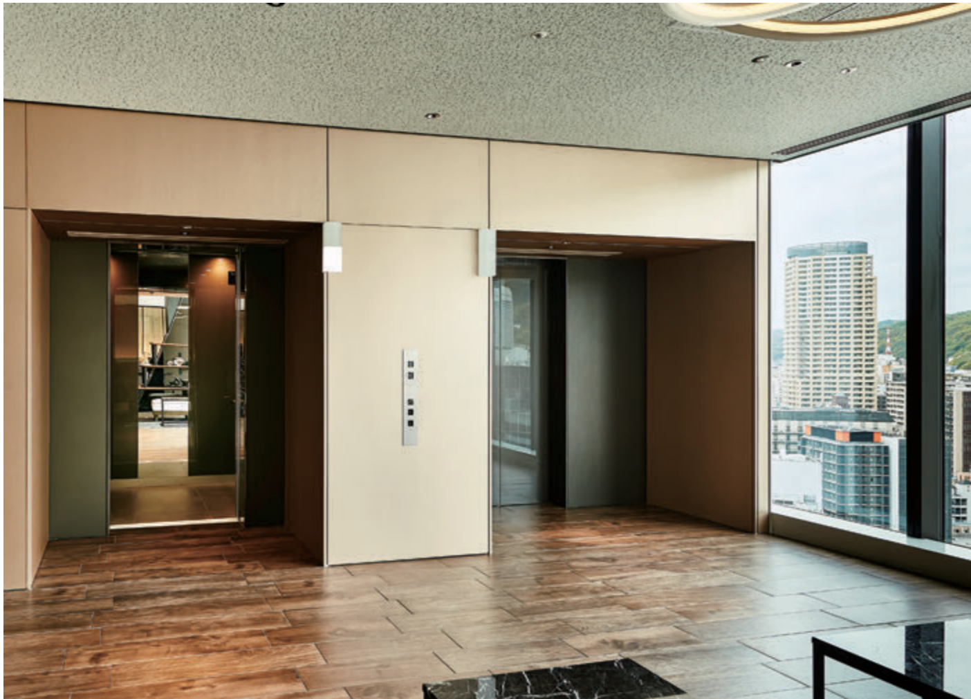
15-person passenger (observation) elevator, lobby floor hall (remm plus Kobe Sannomiya )
