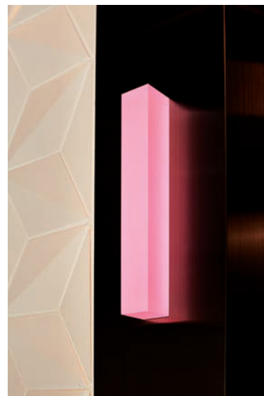
24-person passenger elevator, hall lantern
