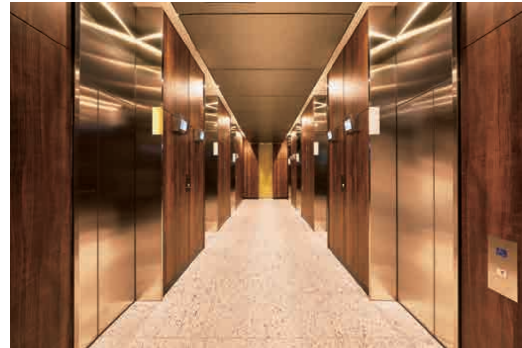
11-person passenger elevator, 1st floor elevator hall
