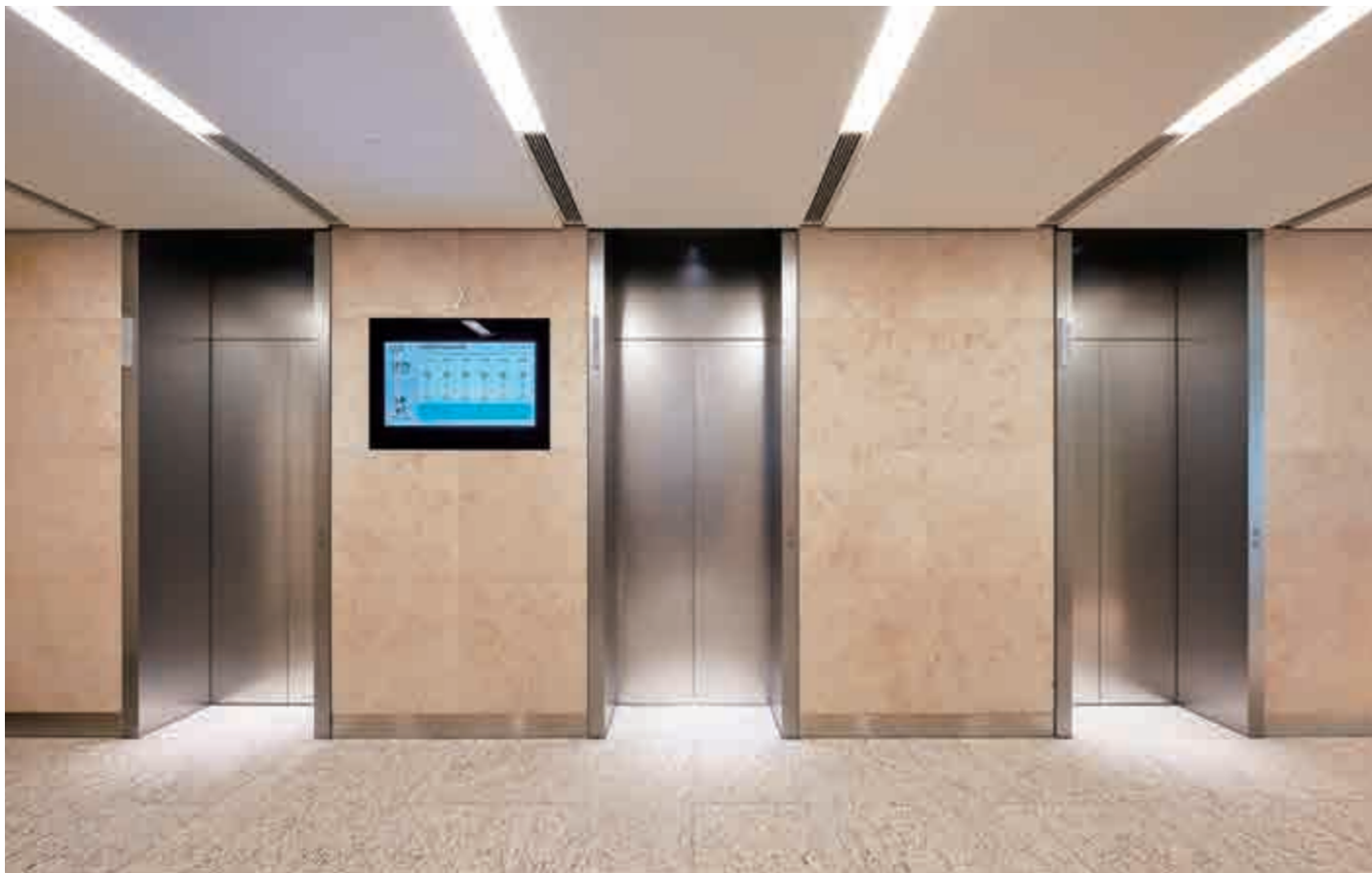
30-person passenger elevator, 2nd floor elevator hall (Mitsui Bussan Building)
