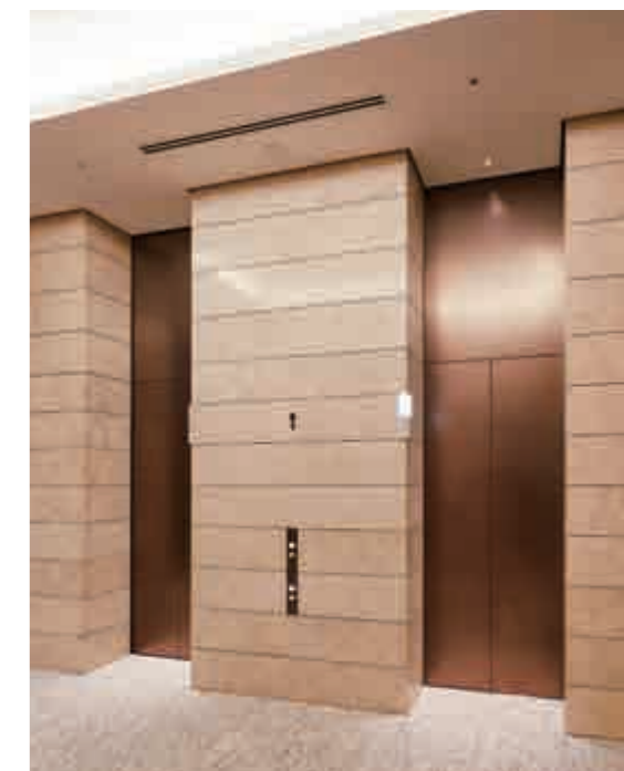
17-person passenger elevator, 1st floor elevator hall (Otemachi One Tower)
