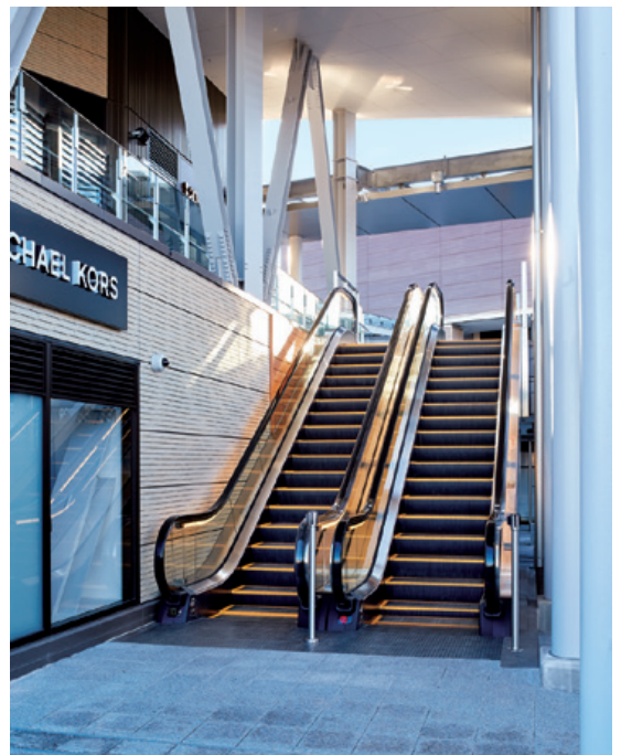
Escalator (Central Court)
