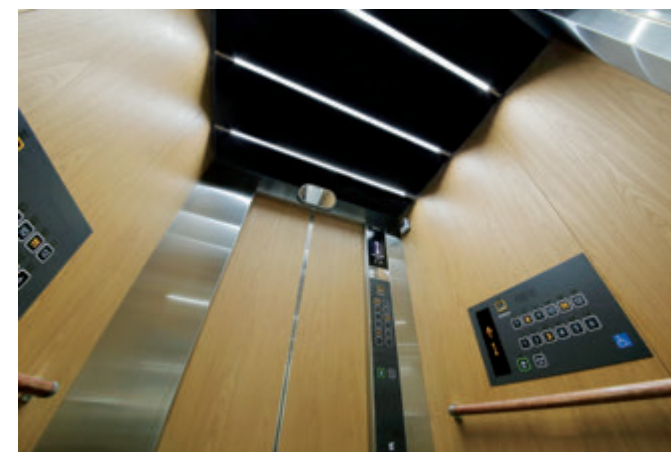
15-person passenger elevator car ceiling
