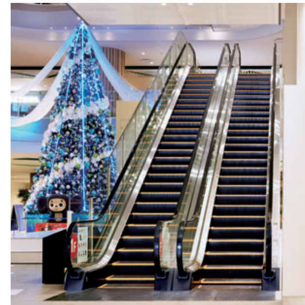
Escalator, 1st floor (Center Court)
