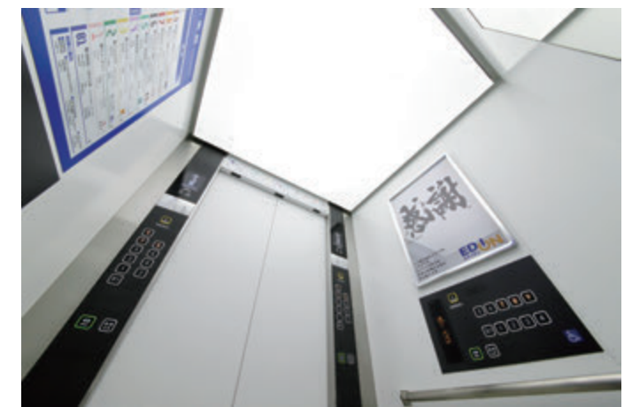
15-person passenger elevator car ceiling
