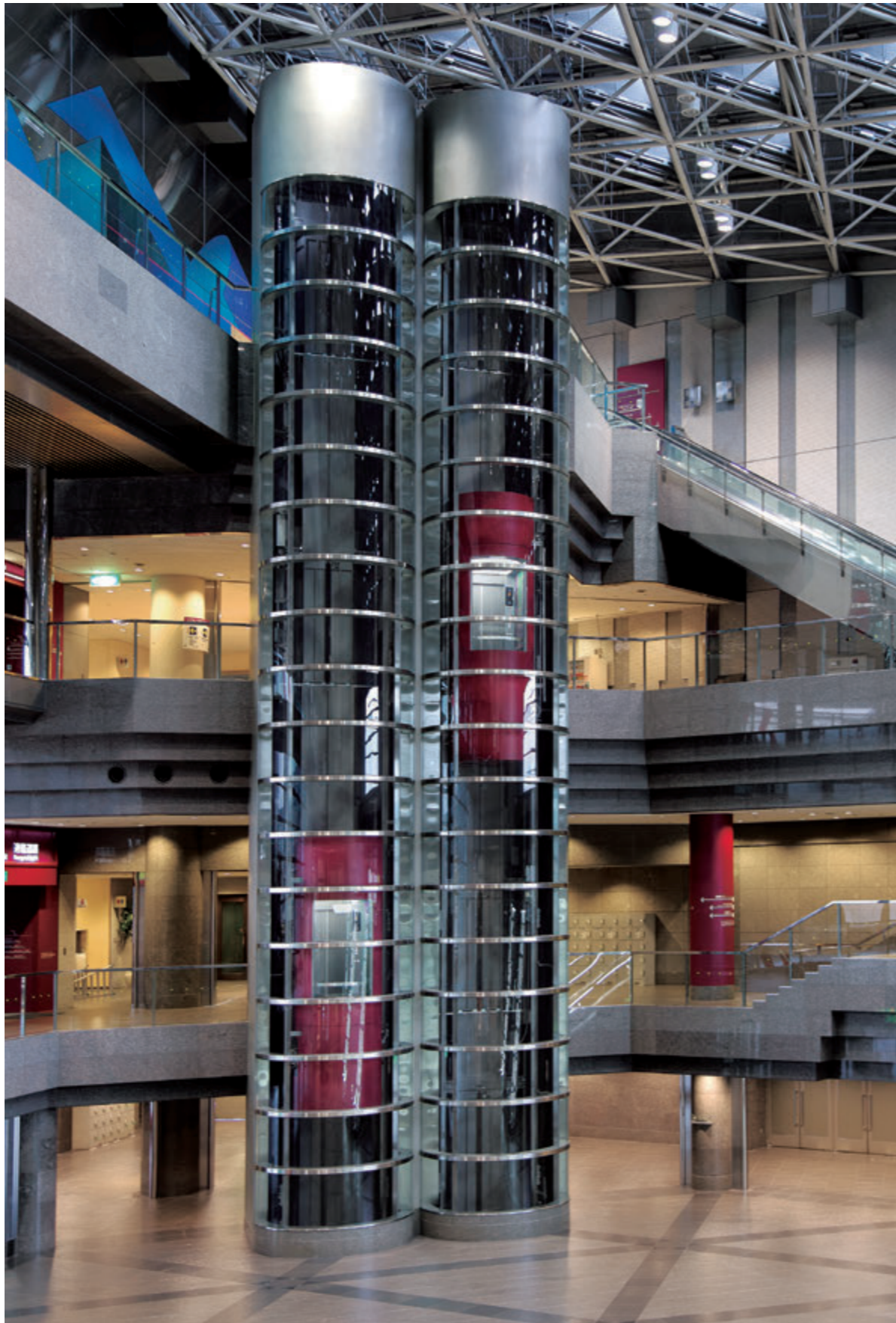
15-person observation elevator car shaft and car
