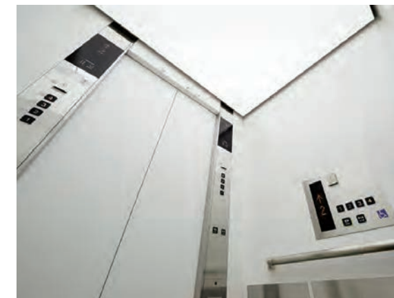
15-person passenger elevator car ceiling
