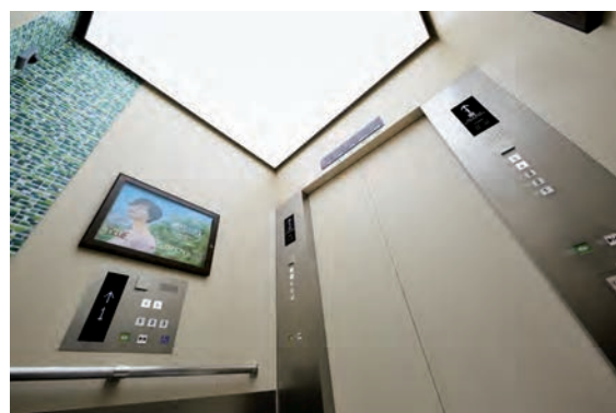
20-person passenger elevator car ceiling
