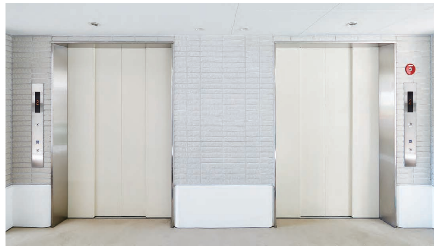
24-person passenger elevator and 26-person passenger (emergency) machine room-less elevator, 1st floor hall
