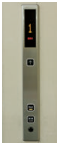
Landing indicator buttons with door open button
