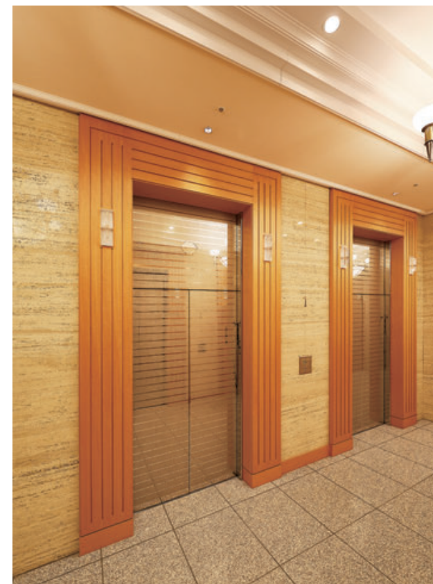
24-person passenger elevator, 1st floor hall (renewal leveraging original landing doors and jamb)
