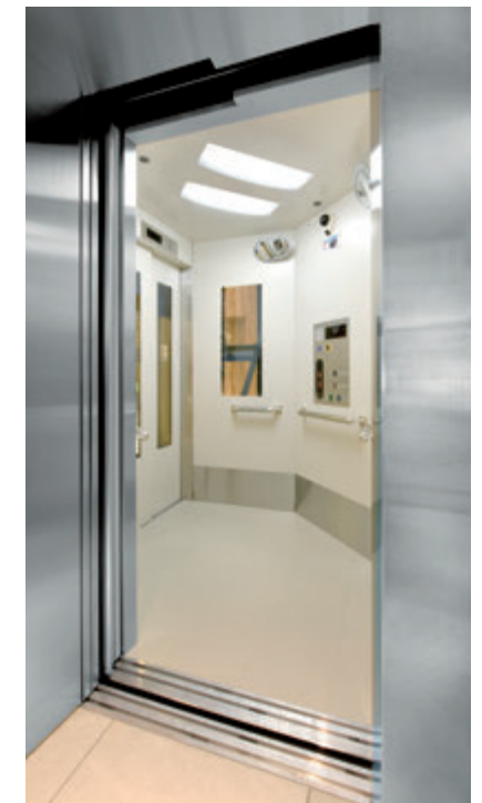
11-person observation elevator car (JR Chiba Station)
