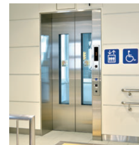
15-person passenger elevator (Chiba Urban Monorail Chiba Station connecting passage)
