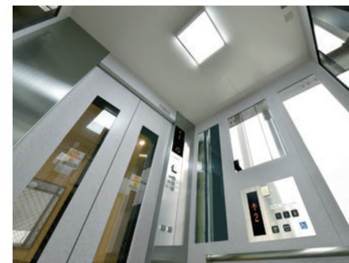
15-person passenger elevator car ceiling (Chiba Urban Monorail Chiba Station connecting passage)
