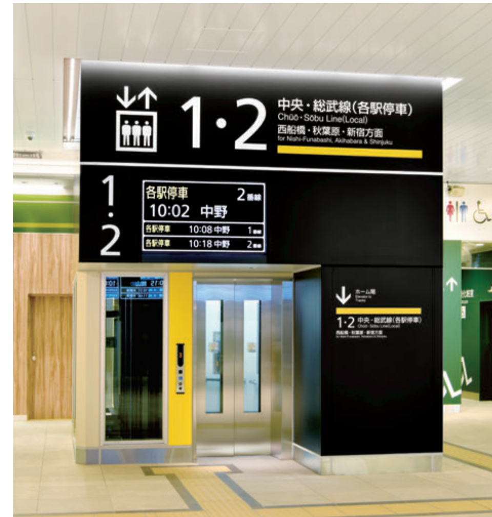
11-person observation elevator, ticket gate floor landing (JR Chiba Station)
