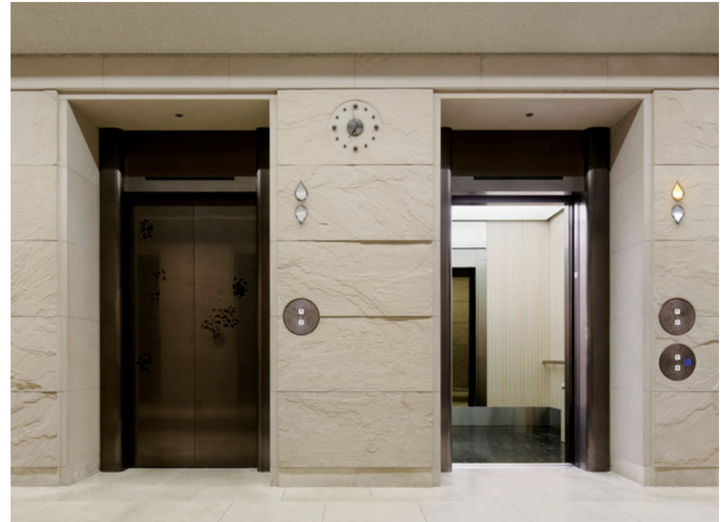
Passenger elevator, 1st floor hall (after renewal, renewal leveraged existing landing doors and jamb)
