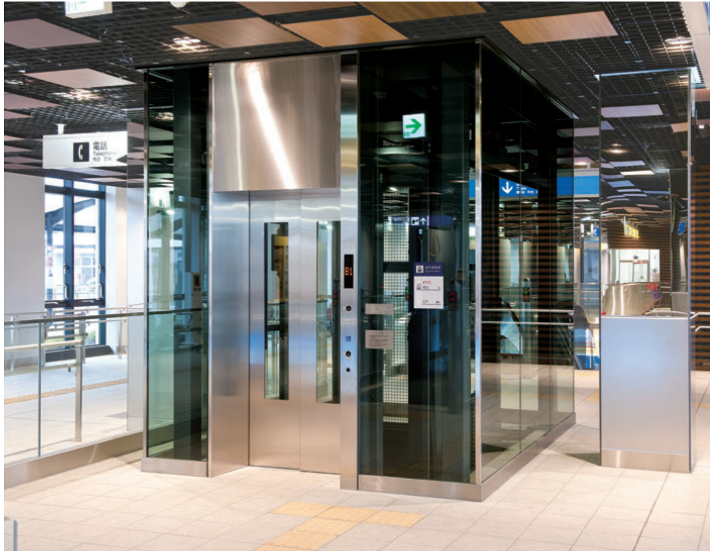
13-person passenger elevator (Arai Station ticket gate floor)
