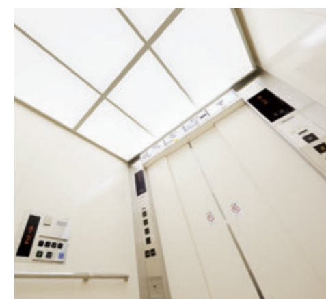
30-person passenger elevator car ceiling
