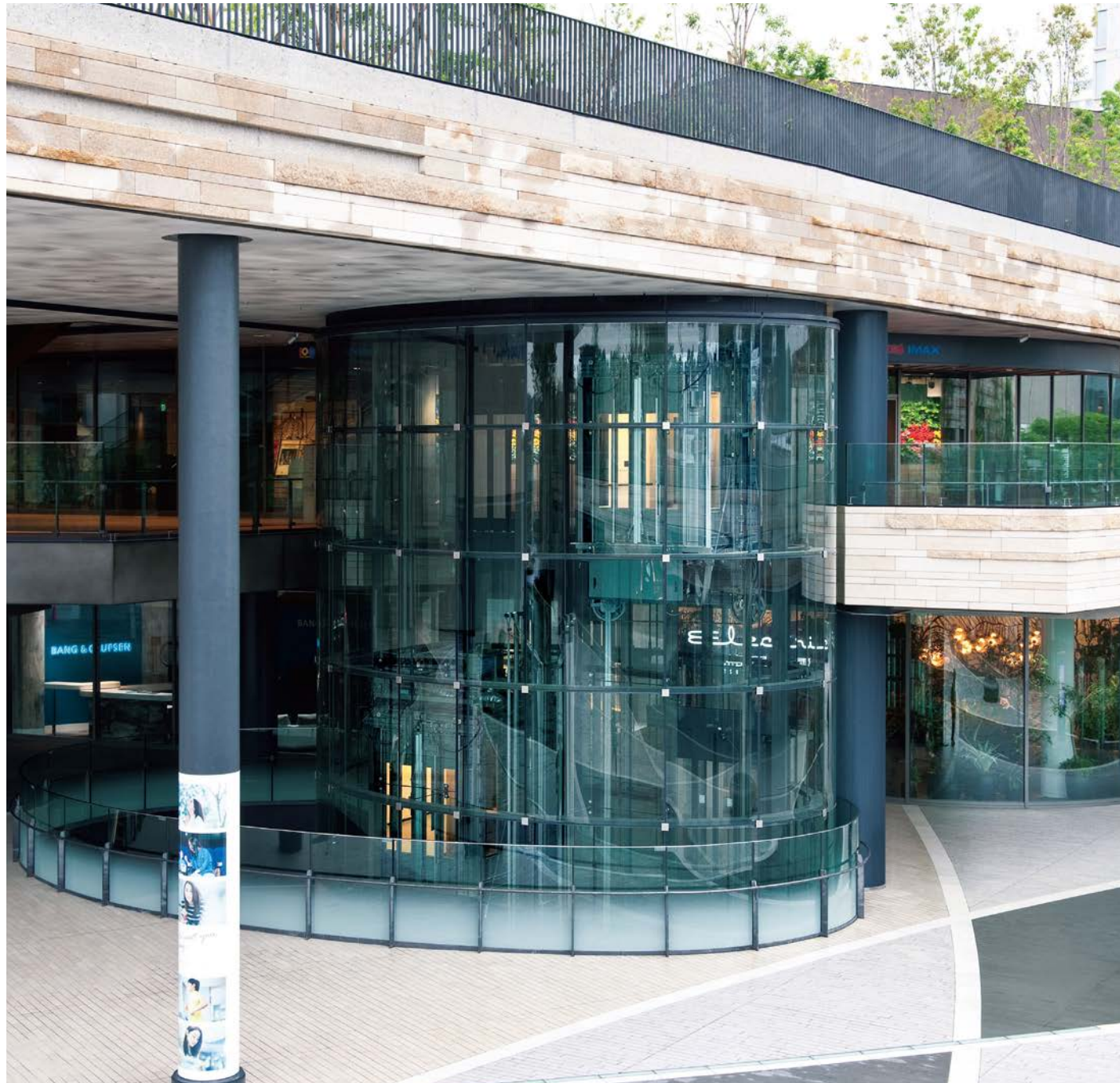
Observation elevator shaft
