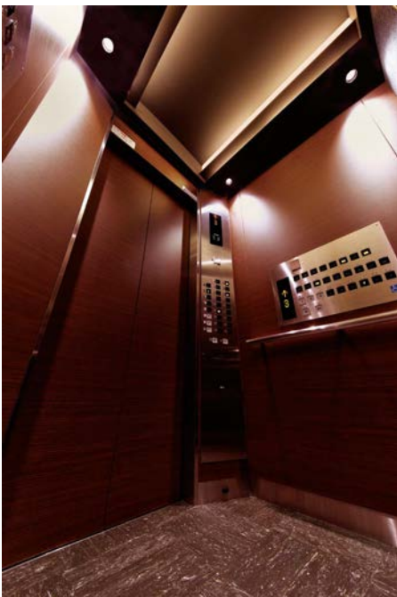
11-person passenger elevator car
