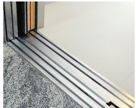
"Gap-free elevator design" fills gap between building and elevator
