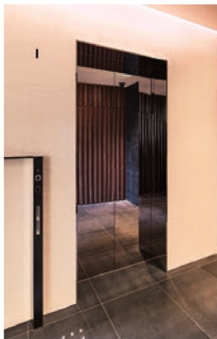
13-person passenger elevator, 1st floor hall
