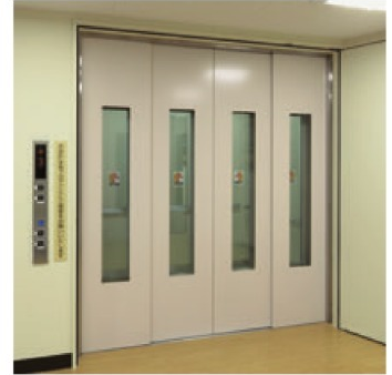
30-person passenger elevator, 3rd floor landing
