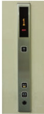
Landing indicator buttons with door open button
