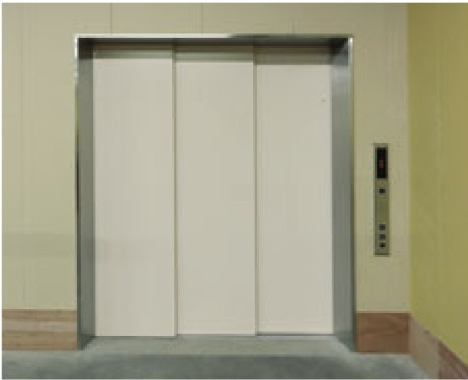
30-person passenger and freight elevator, 1st floor landing
